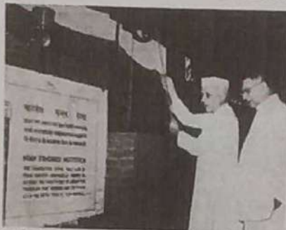
Mr. Nehru laying the foundation stone of the building of the Indian Standards Institution in Delhi on Saturday. Mr. V. V. Kishanbhai is also in the picture.
